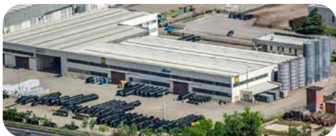
Production Facility - Imola (BO)
