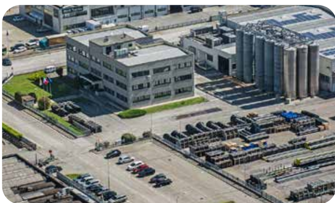
Production Facility - Castel Guelfo di Bologna (BO)
